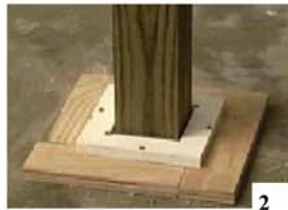
2. THE SECOND STEP IN THE INSTALLATION PROCESS IS TO INSTALL THE SQUARING BLOCKS TO THE FLOOR AND TO THE HEADER. THIS MAY BE DONE USING STAPLES, NAILS, SCREWS, OR ADHESIVE. THE SQUARING BLOCKS WRAP AROUND THE STRUCTURAL POST AND ACT AS AN INDEXING BLOCK FOR THE COLUMN SO BE SURE THAT THEY ARE SQUARE AND PLUMB AT THE TOP AND BOTTOM.
