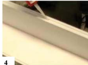
4. NOW YOU NEED TO APPLY ADHESIVE TO BOTH EDGES OF THE REMAINING HALF OF THE COLUMN
