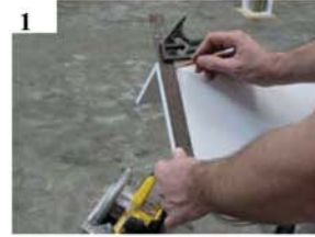
1. THE FIRST STEP IS TO CUT THE COLUMN TO THE DESIRED LENGTH. THIS CAN BE DONE USING A SKILL SAW.
