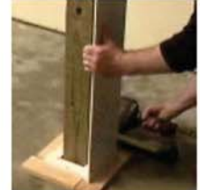
3. NEXT INSTALL ONE HALF OF THE COLUMN AND ATTACH IT TO THE SQUARING BLOCKS AT THE TOP AND BOTTOM.
