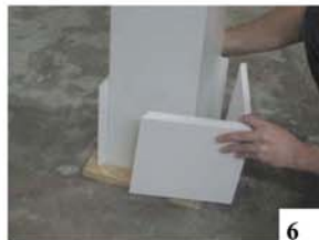
6. NOW YOU NEED TO ATTACH THE COLLARS TO THE SHAFT. DO THIS BY WRAPING THE COLLARS AROUND THE SHAFT AT THE TOP AND BOTTOM AND FASTENING THEM TO THE SHAFT AS WELL AS FASTENING BOTH HALVES TOGETHER AT THE CORNERS. PLEASE NOTE THAT IF YOU ORDERED A SPECIAL CAP IT IS INSTALLED THE SAME WAY AS A COLLAR.
