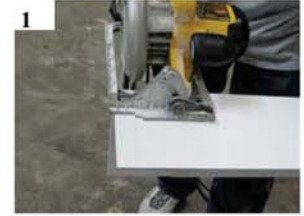
1. THE FIRST STEP IS TO CUT THE COLUMN TO THE DESIRED LENGTH. THIS CAN BE DONE USING A SKILL SAW.
