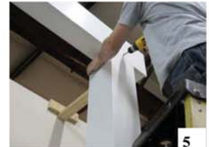
5. NEXT LINE UP THE OTHER HALF OF THE COLUMN AND FASTEN IT TO THE FIRST HALF. FASTEN THE COLUMN ON BOTH EDGES AS WELL AS ATTACHING IT TO THE SQUARING BLOCKS. WE RECOMMEND FASTENING THE COLUMN EVERY 8 TO 10 INCHES USING 1-1/4" STAPLES.
