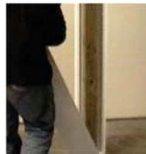
5. NEXT LINE UP THE OTHER HALF OF THE COLUMN AND FASTEN IT TO THE FIRST HALF. FASTEN THE COLUMN ON BOTH EDGES AS WELL AS ATTACHING IT TO THE SQUARING BLOCKS. WE RECOMMEND FASTENING THE COLUMN EVERY 8 TO 10 INCHES USING 1-1/4" STAPLES.
